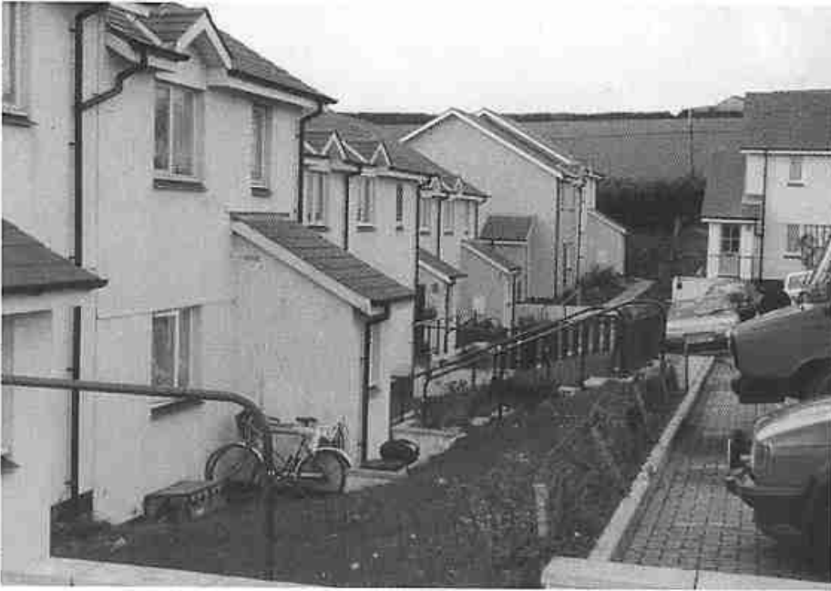
Affordable housing at Greenbanks Close
